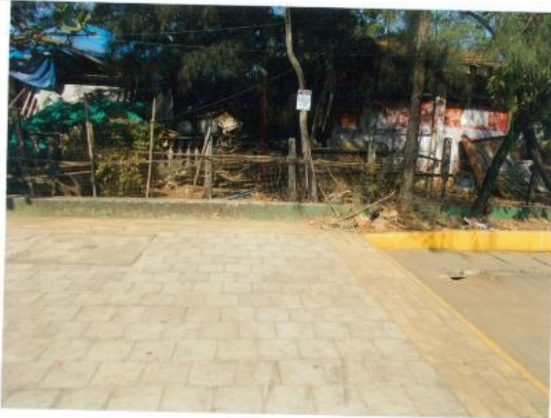
Space after crossing Foot Over bridge at Income Tax Office leading to EDC Patto Panaji
