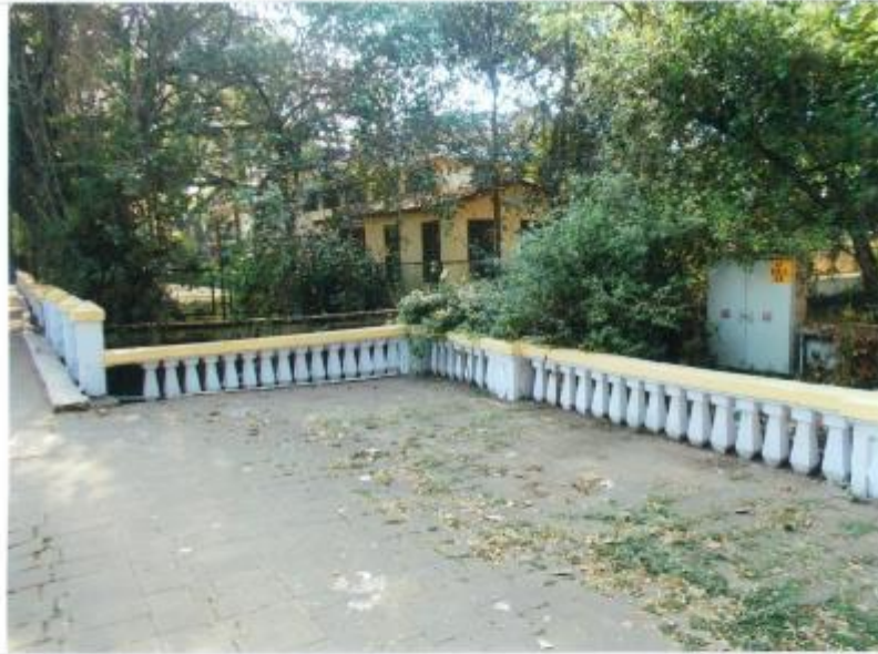
Opposite Bal Bhavan (wider Footpath on D.B. Road Panaji Goa
