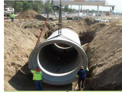
Laying of Storm Network
