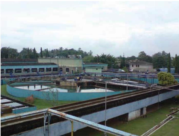
Ambatale Water Purification Plant in Colombo.
