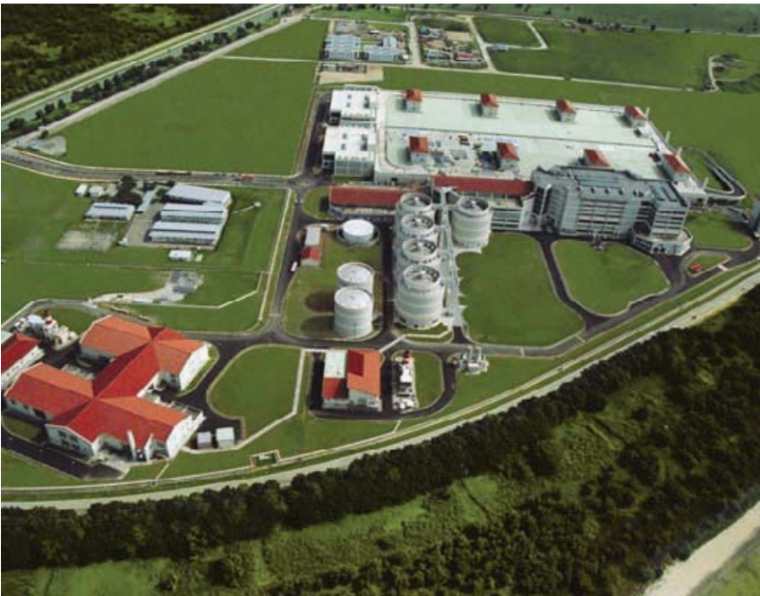
Figure 9 The Changi Water Reclamation Plant
