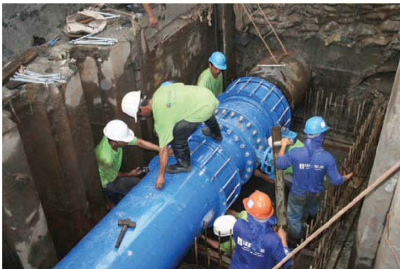
Contractors at work during an interconnection activity in Sta. Mesa, Manila.
